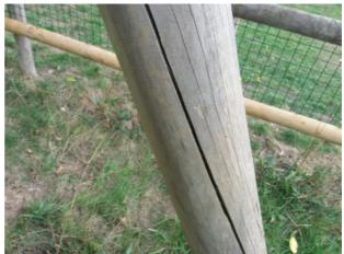
All timber posts have a number of splits/shakes or air cracks and this may affect the stability or allow water ingress which will accelerate the rotting process Finding:
