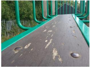
Finding: The timber platform is rough and worn
