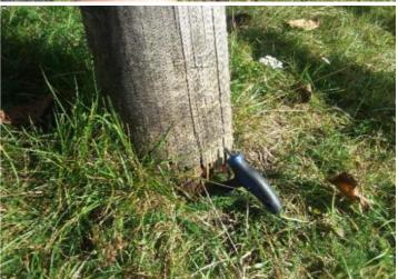
**Finding:** There are areas or parts of the timber support post **Action:** Replace all affected timbers on the structure that have rotted
