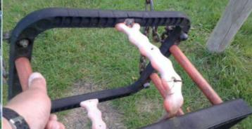
Finding: The swing seat frames are corroding
