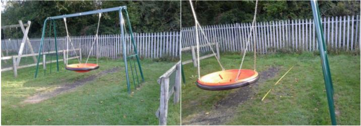
**Finding:** The edge of the impact area is less than 1.5m from **Action:** Monitor - No remedial work recommended the fence; BS EN 1176, Annexe A; we consider this to be a low risk finding and no remedial action is required
