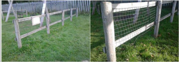
**Finding:** The mesh has been damaged and sharp wires are **Action:** Repair or replace the item protruding
