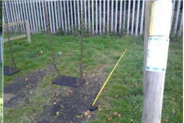
**Finding:** The edge of the impact area is less than 1.5m from **Action:** Monitor - No remedial work recommended the fence; BS EN 1176, Annexe A; we consider this to be a low risk finding and no remedial action is required
